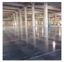
The floor of the distribution centre, belonging to a well known supermarket chain Masoutis S.A. in Greece, was built by Eurolit using Laser Screed construction to meet at least with Line 4 of the DIN 18202 – the strictest DIN free movement specification. CG's involvement in the project was to use their patented Laser Grinder® technology to grind the narrow aisles to a tolerance suitable for the VNA
